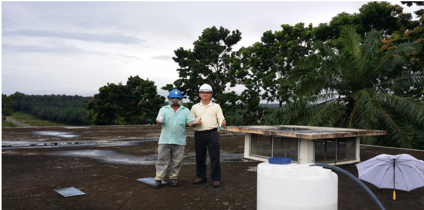
Rosun DW-1 Dosing by gravity flow on clarified water tank
